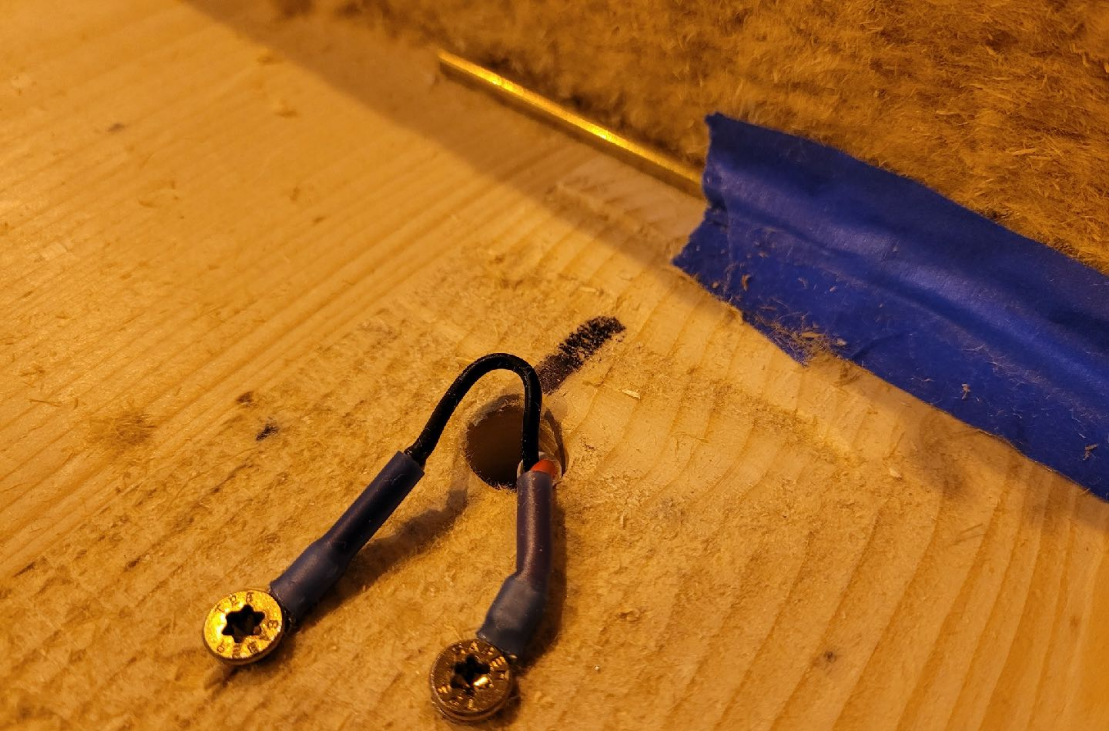
U-Maine Installs Sensors in Roof + Wall Assemblies
