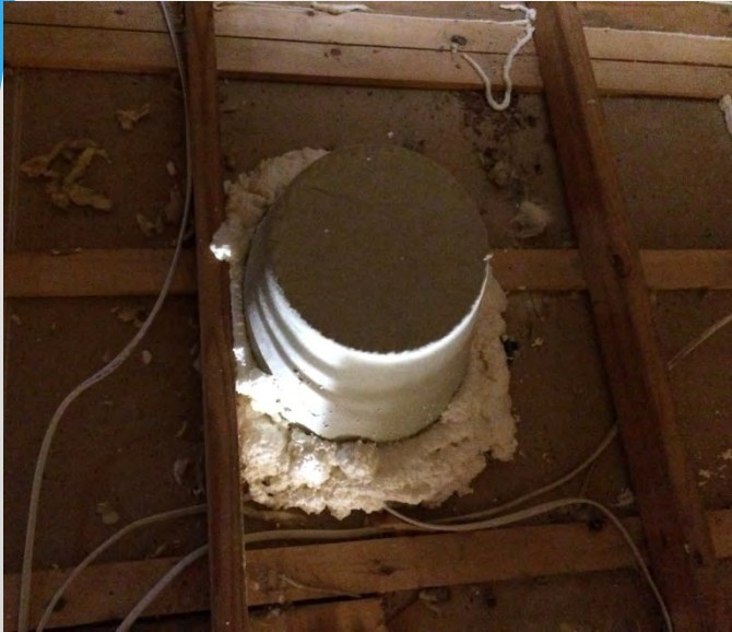
Mineral wool covers over recessed can lights, sealed to attic floor
