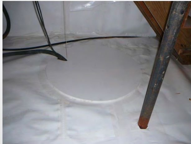
Vapor barrier and sealed cover over old cistern
