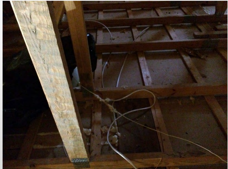
Utility penetrations sealed at attic floor
