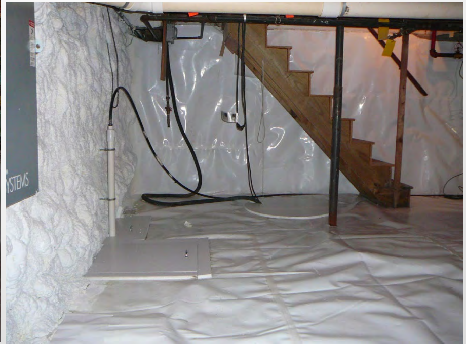
Vapor barrier and sealed cover over sump
