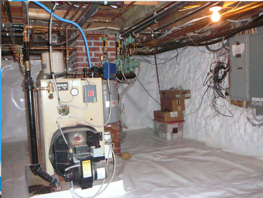
“Fan in a Can” for positive pressure in basement
